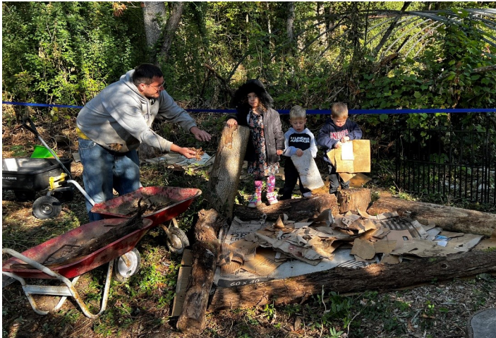
Willow Joy, Tate and Crew lay the foundation for the new flower bed.
