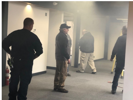
Final test for Falcon Pod with building inspector for electric, H-Vac and fire alarm with real smoke.
