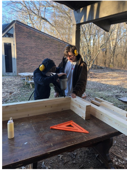
Aydon P and Nathan build a bench.
