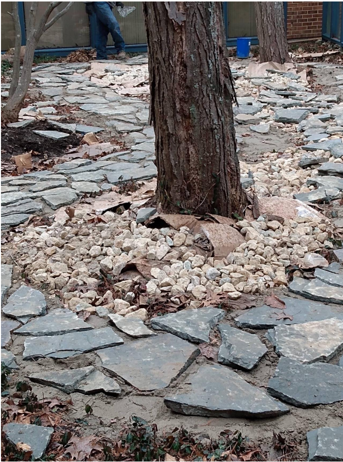
The Eagles are eagerly anticipating the use of their Quiet Outdoor Garden. The Wings are working feverishly to complete a Pennsylvania Bluestone paving around our gorgeous Japanese Maple tree. So far the Wings have carried about three tons of stone and two tons of sand. More pictures will follow when work is complete.
