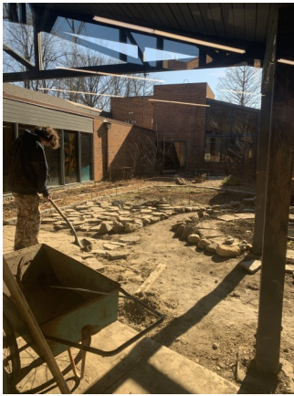
Dominic working on the new Wing and Falcon Courtyard.
